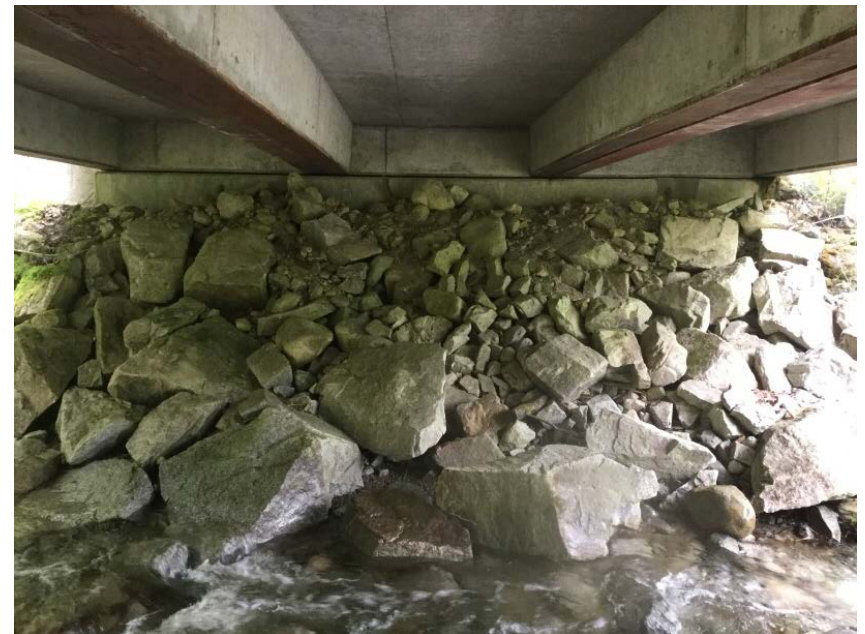
Left Bank Abutment when facing downstream
